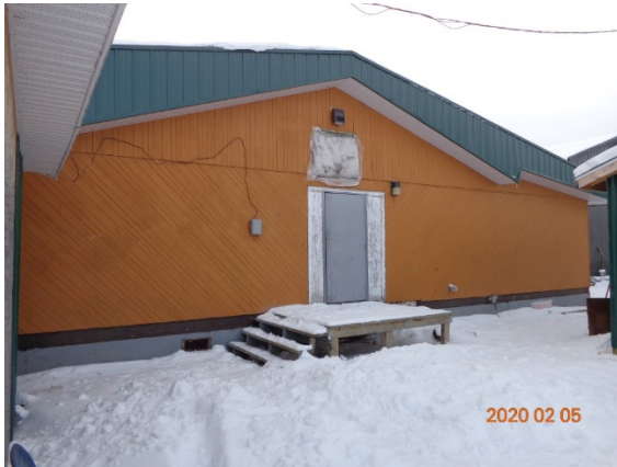
A7 – Back service door
