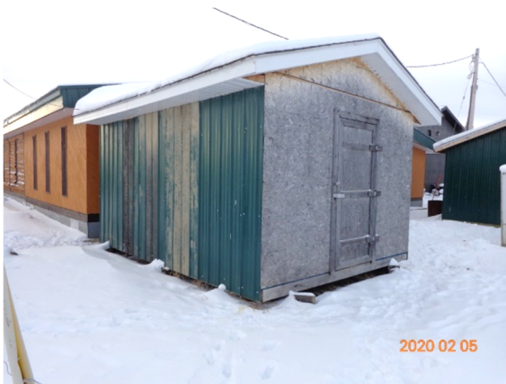
A29 – East cold storage shed
