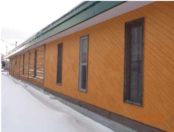
A9 – Exterior windows & finishes
