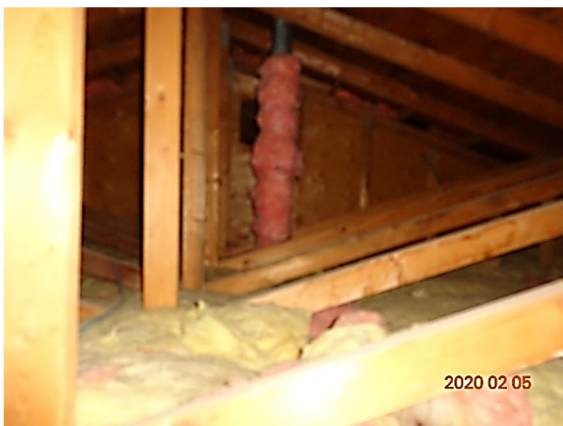
A11 – Attic & roof structure
