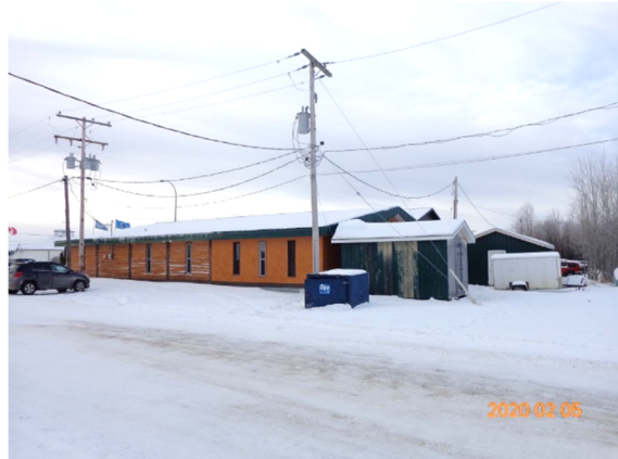
A2 – Friendship Centre & rear storage buildings
