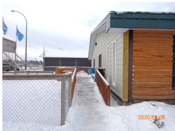
A6 – Ramp up to deck at main entrance
