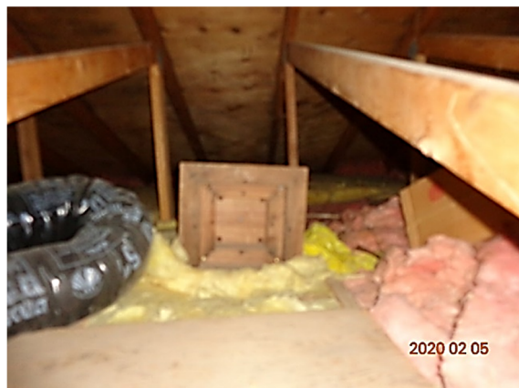
A12 – Attic & roof structure
