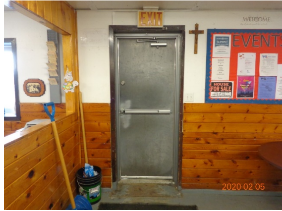
14 – Interior view of main entrance
