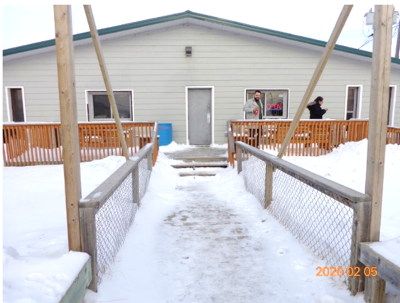
A5 – Stair & deck to main entrance
