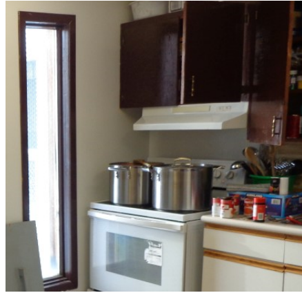
M8 – Kitchen range exhaust hood ducted to outdoors
