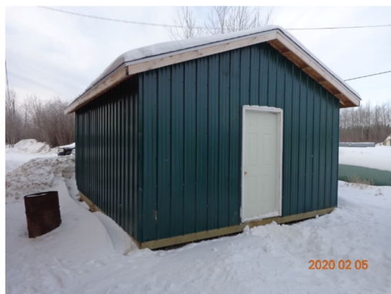
A30 – West cold storage shed
